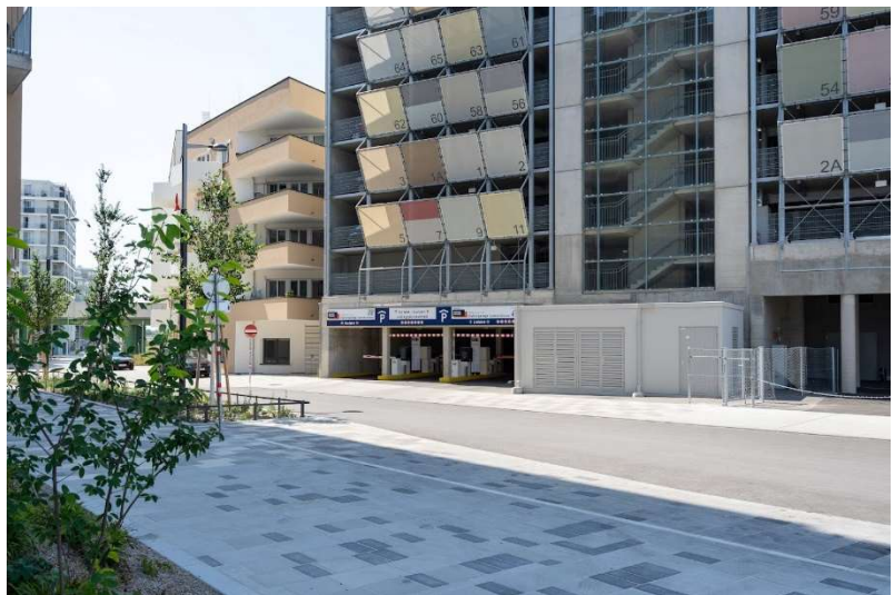
The garage is located at the end of the street (address: Ilse-Buck-Straße 23).
